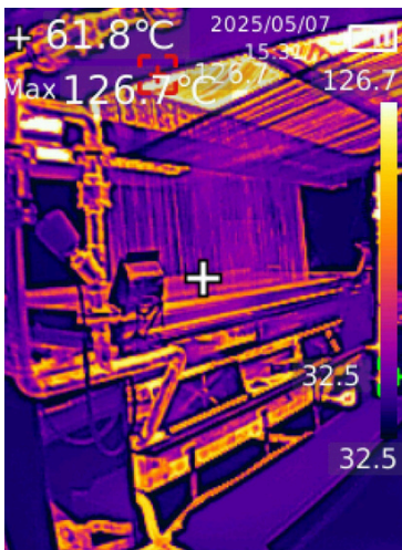
Image 12: Thermal Image of Sizing Unit
